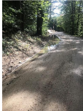
Loose soil and gravel and ponding evident near new construction on Stockbridge Corner Rd.
