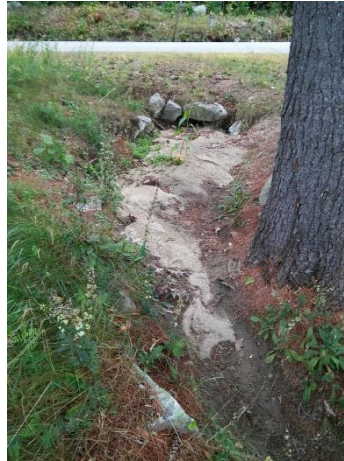
Significant sediment erosion of road ditches and parking area on both hillslopes leading to Merrymeeting River.
