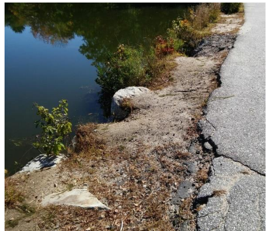
Underwater stone culvert connects Mill Pond with the Merrymeeting River. Surface erosion evident.
