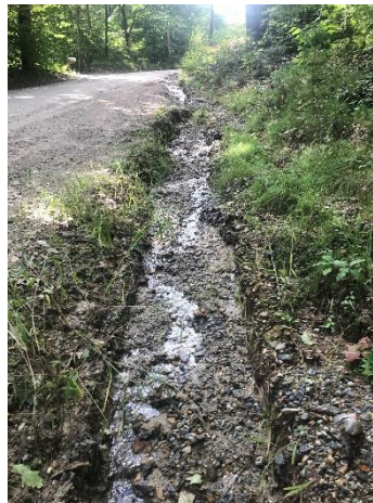
Deep gully formations in road shoulders and ditches along Stockbridge Corner Rd, leading to a tributary of Coffin Brook.
