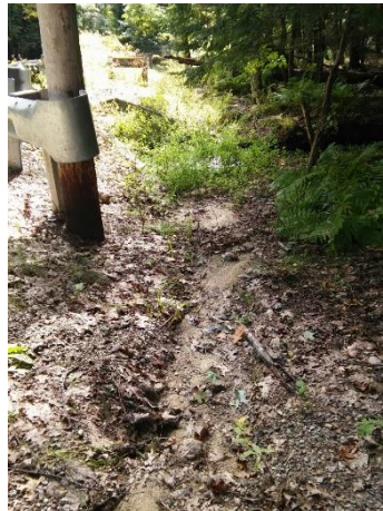
Significant road surface and ditch erosion evident on Horne Rd leading to a tributary of Coffin Brook.
