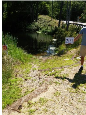
Road runoff forming rills and gullies at Merrymeeting Rd bridge at outlet to Marsh Pond.
