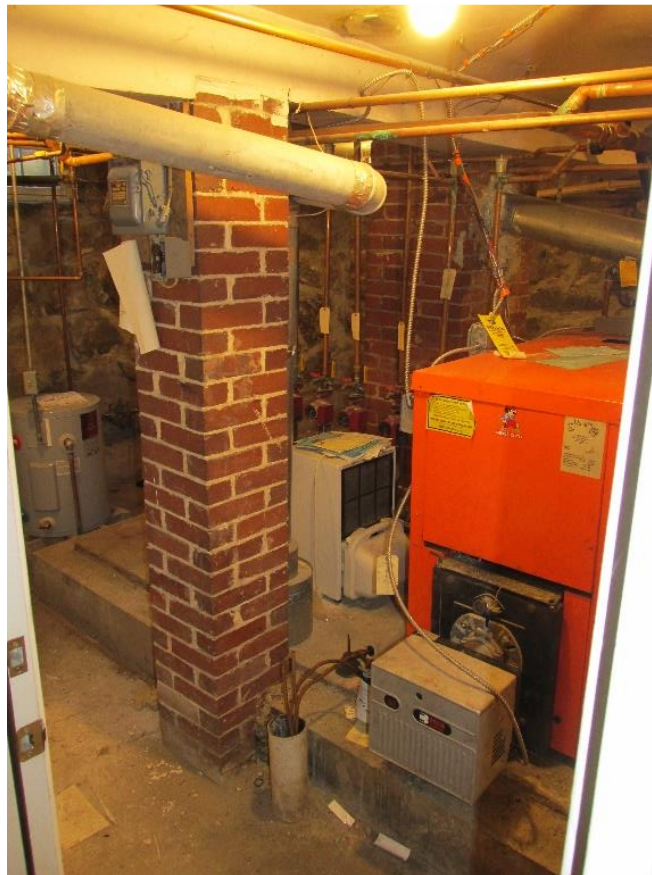
Town Hall Boiler Room
