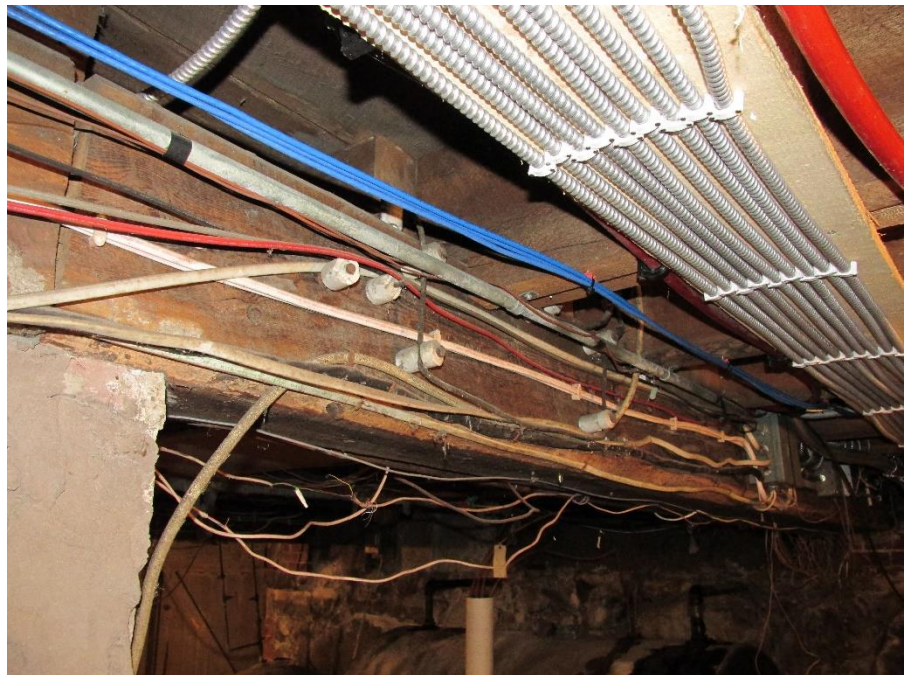
Town Hall Basement - Variety of Vintage Conductors
