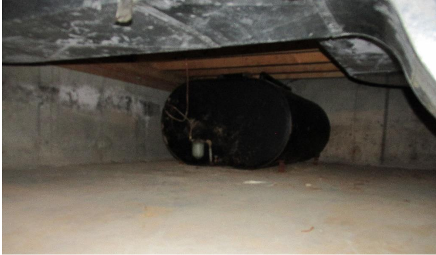
Library Crawl Space - Fuel Oil Tank
