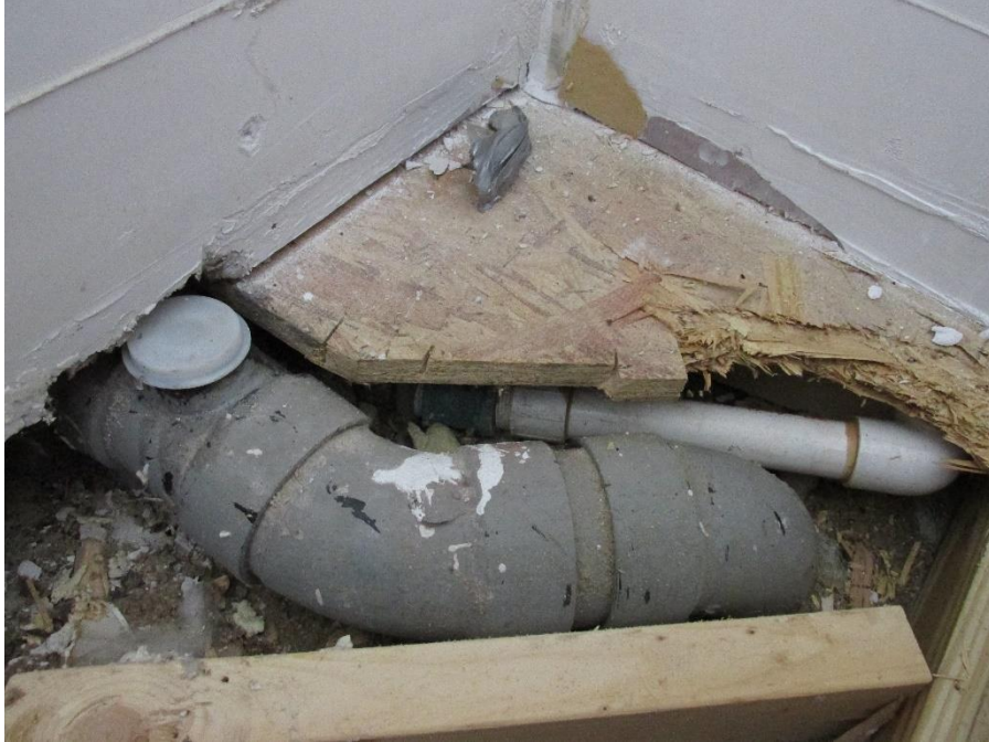
Fire Station Plumbing - Sanitary Main Vent
