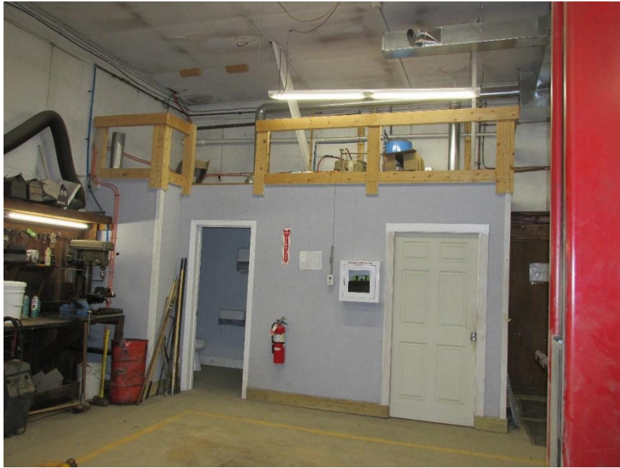
Public Works Equipment Bays - Toilet Rooms
