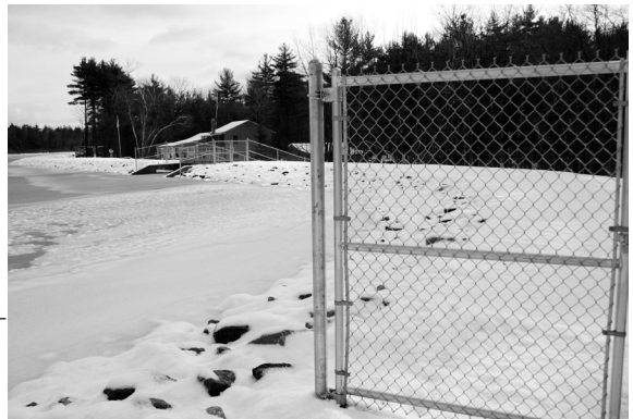
March's Pond Dam
