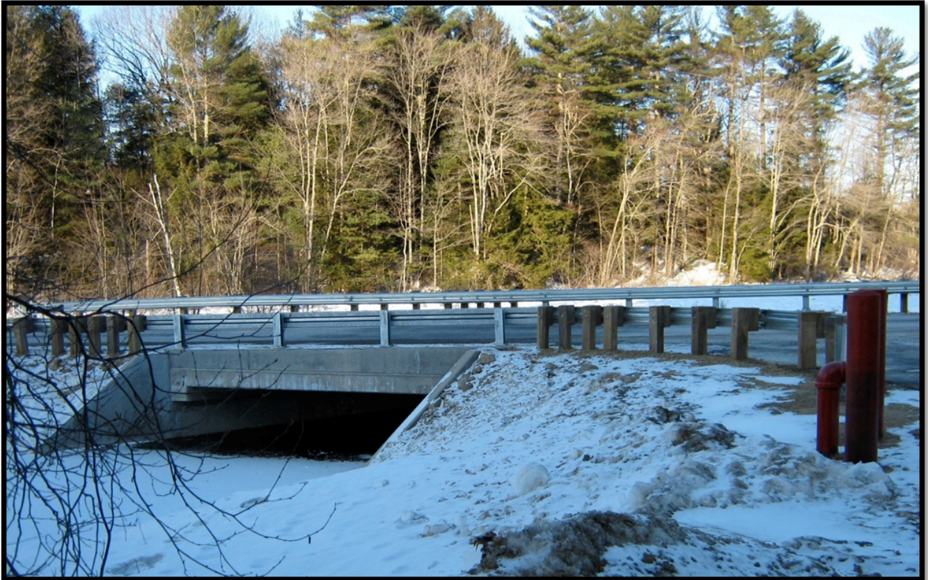
Davis Crossing Road new culvert installed December 2009
